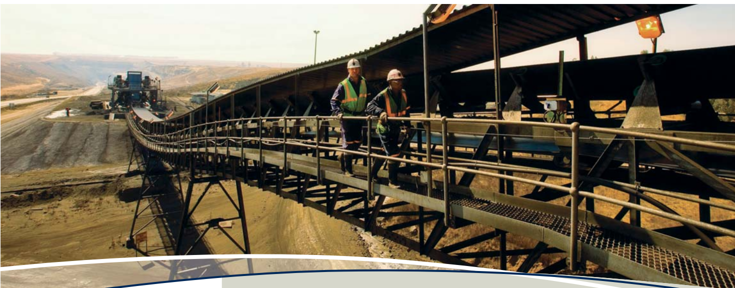
Sasol Mining, in partnership with our BEE partner, Ixia Coal, delivered a remarkable 12% improvement in productivity.
